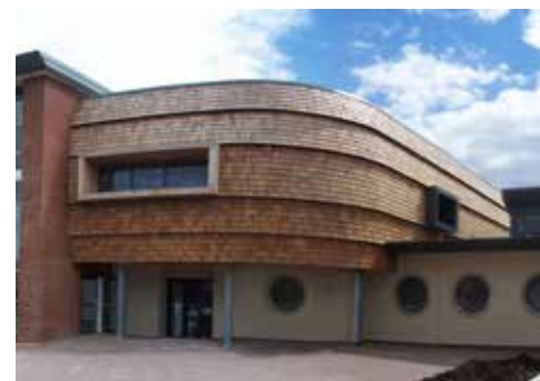
Primary School, Swansea
