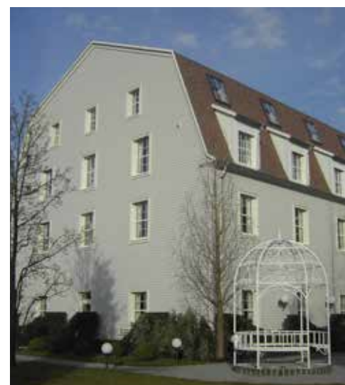
Bell Rock Hotel, Europa-Park External timber cladding prior to coating FR Specification: WPA Type INT2 (Humidity resistant)
